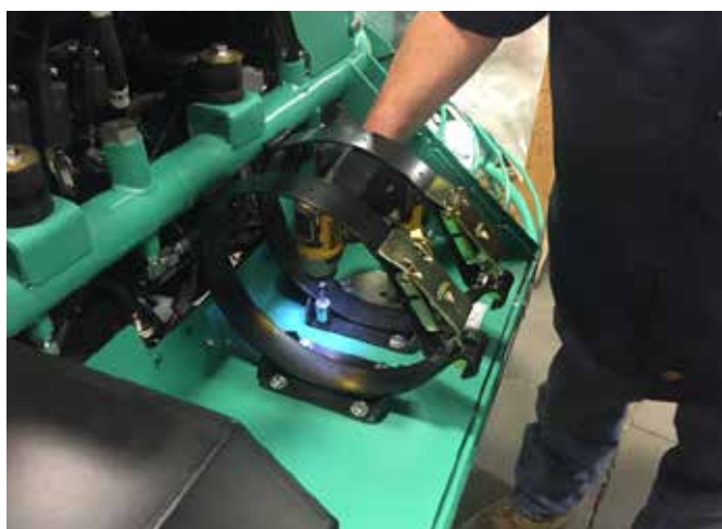
Figure 32. Reattach LPG Tank Straps
