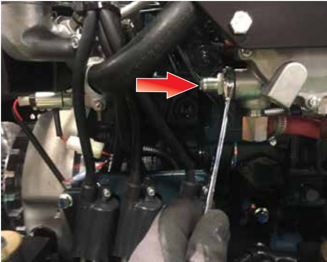
Figure 17. Straight Fitting Removal
